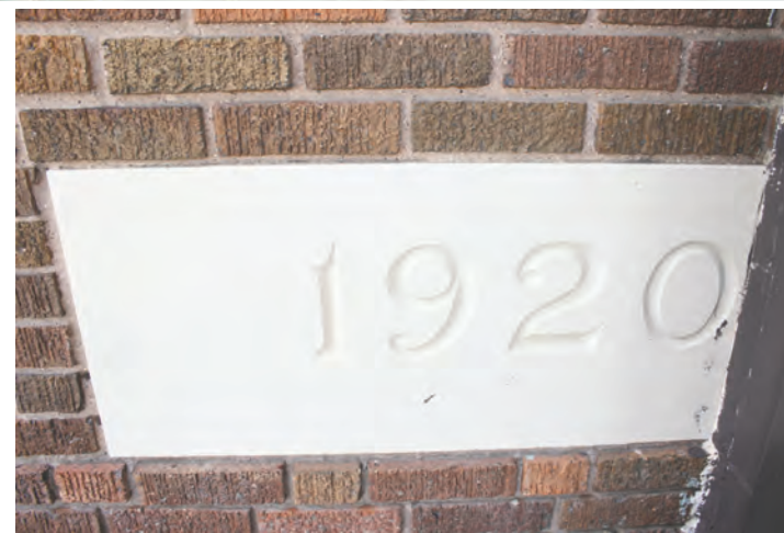
The Eagle Grove High School cornerstone is located on the right side of the center doors on the south side of the building. This is the original cornerstone despite how clean and new it still appears. Photo by Kim Demory
